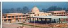
Terminal space including all sorts of facility to tackle sudden peaking of demand
