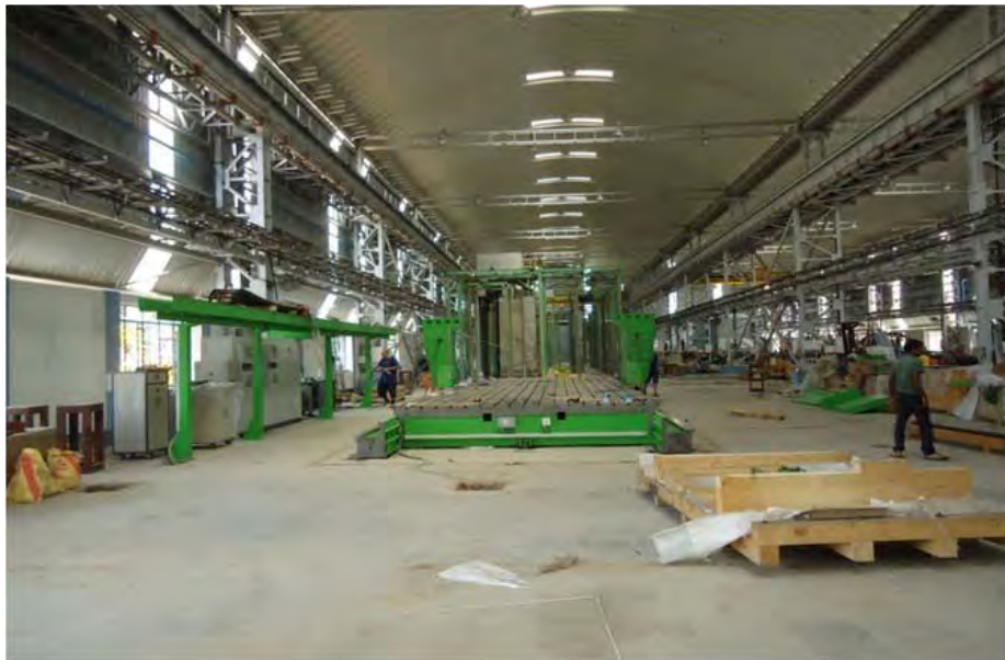
RCF Budge Budge – Plant & Machinery under installation and commissioning.
